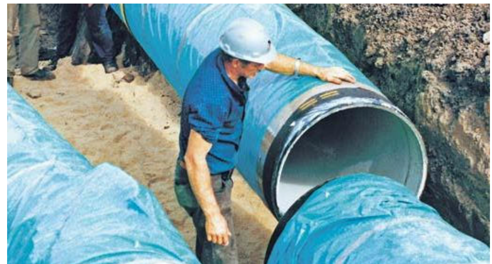
Lubrication of pipe spigot prior to jointing
