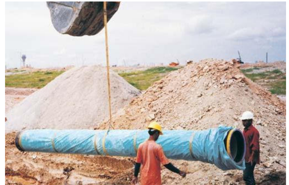
Sleeving pipe with SuperTYT polyethylene sleeving at Kuala Lumpur International Airport
