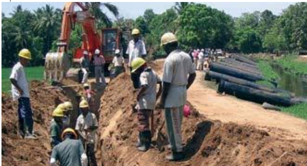
Pipeline construction in Sri Lanka
