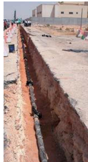
Pipeline construction in Riyadh, Saudi Arabia
