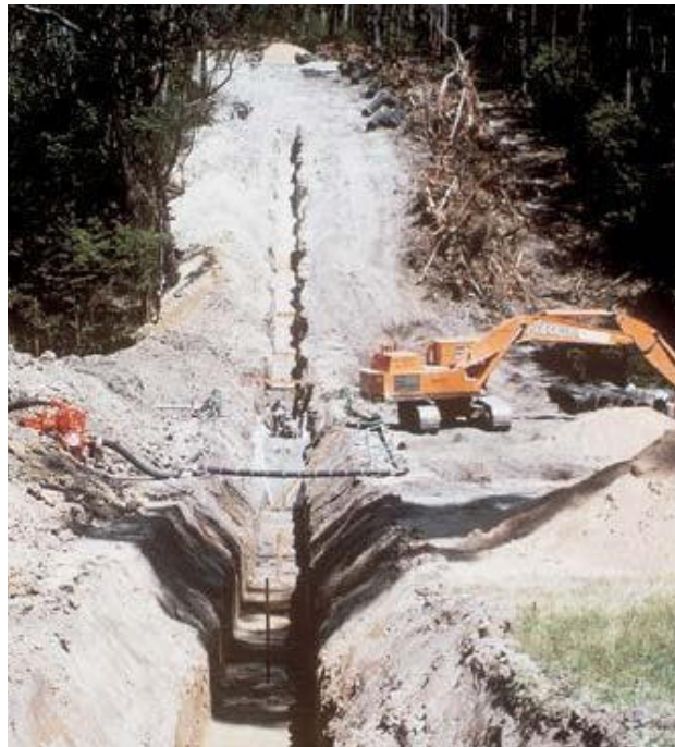
Trench incorporating gradient anchors
